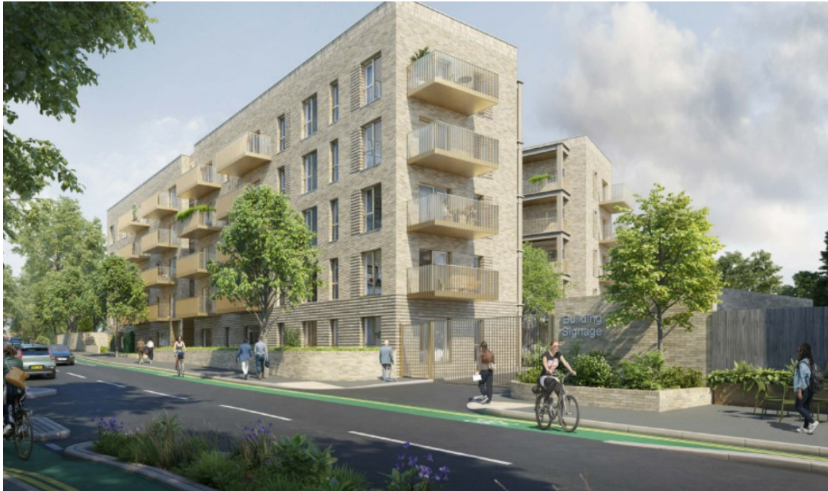
Visual image when looking northwards along Manchester Road
