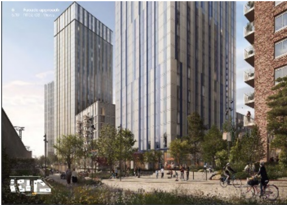
Image of towers 1 and 3 (mid rise buiding in the middle) with along Dulwich Street South
