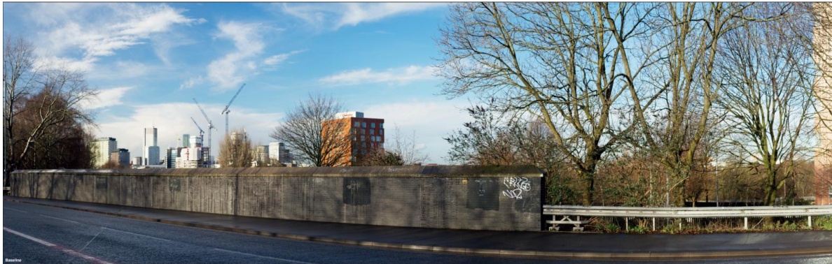
Viewpoint 6 Rochdale Road (Railway Bridge) (existing)
