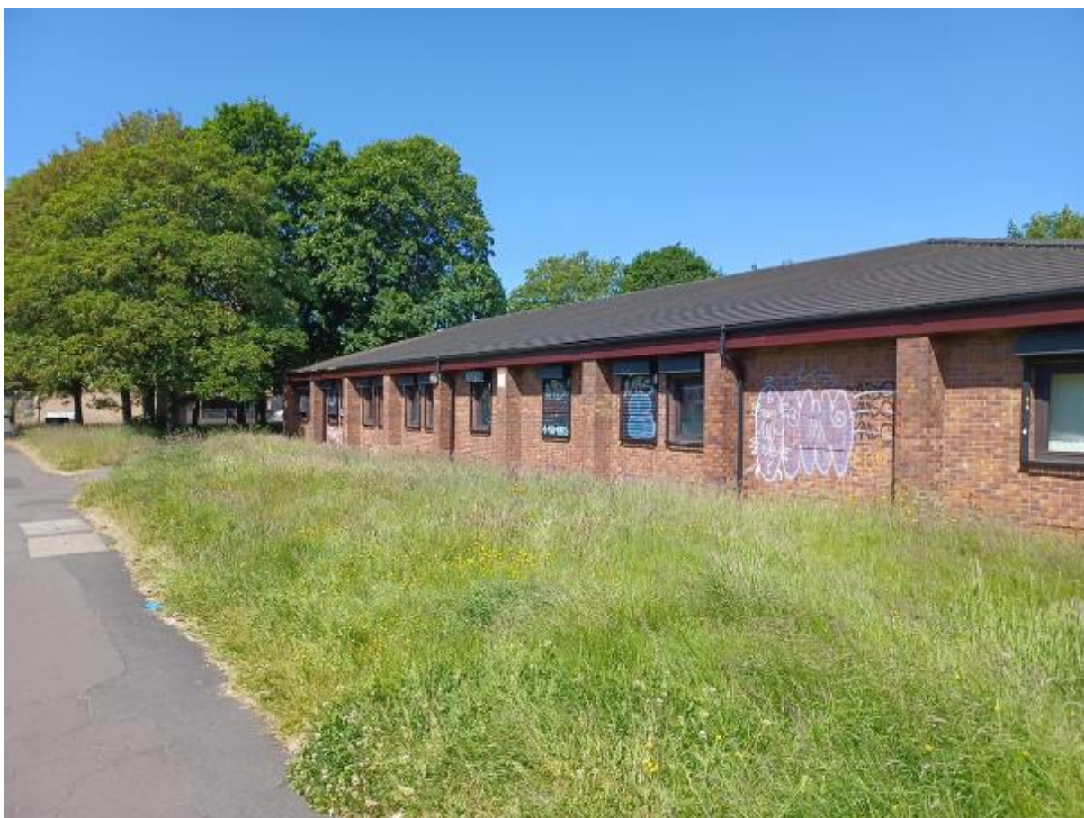
Moss Lane West elevation of existing Probation building
